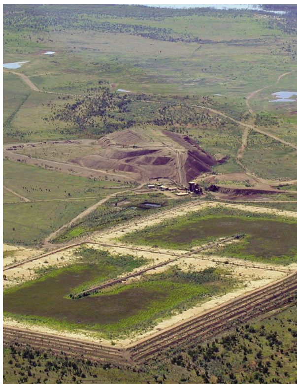
AF709 31/08/2012 Figure 5.6 View looking north over the Bow River alluvial diamond mine processing plant and tailings dams
